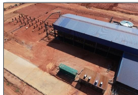
Electrowinning plant extension
