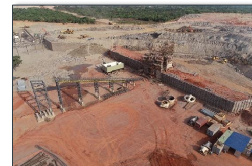
Expanded crusher under construction
