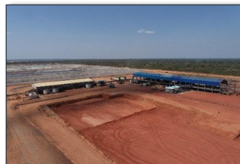
SX/EW plant & expansion groundworks
